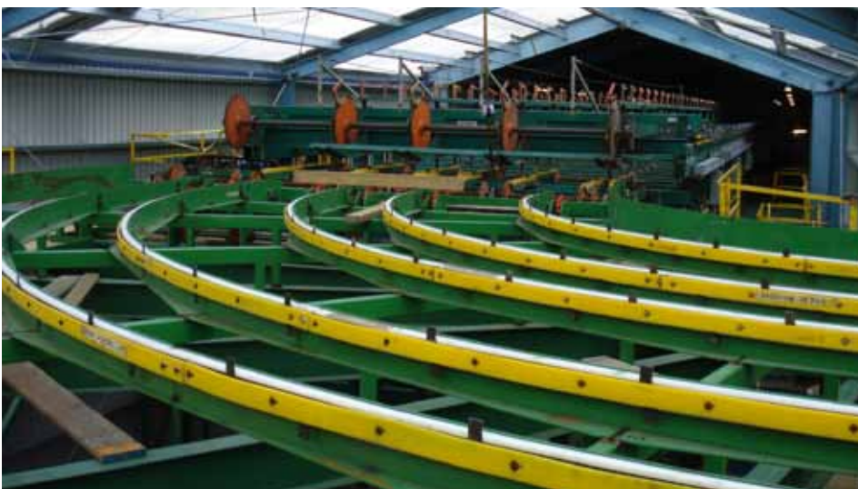
Pictured is one of two 90-degree turn transfers, part of the complement of new equipment that was included to meet the specific requirements for the mill's new layout.
